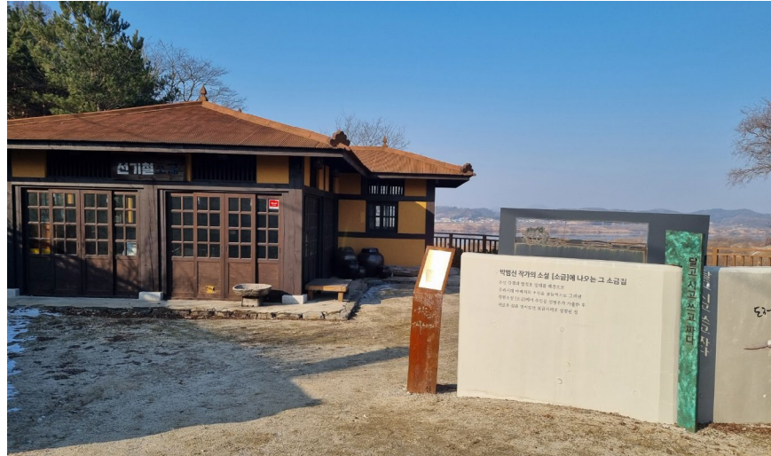
The salt house recreated in Ogyeobong
